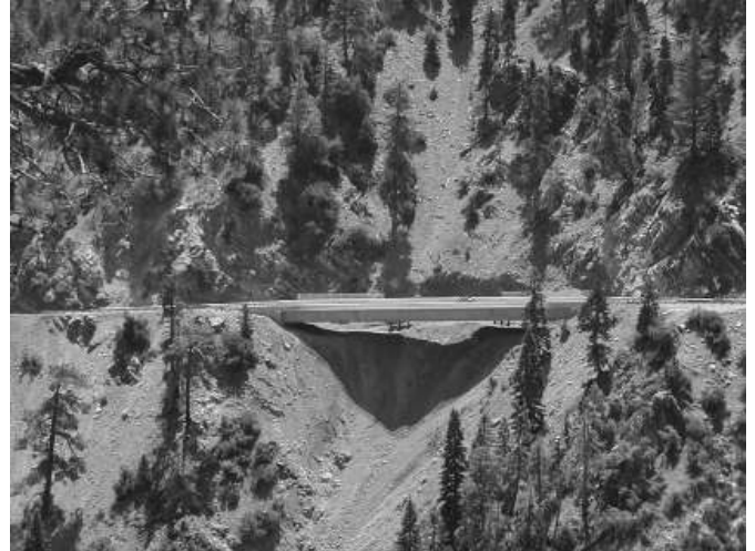
The newly constructed bridge on the Angeles Crest Highway just west of Vincent Gap.
