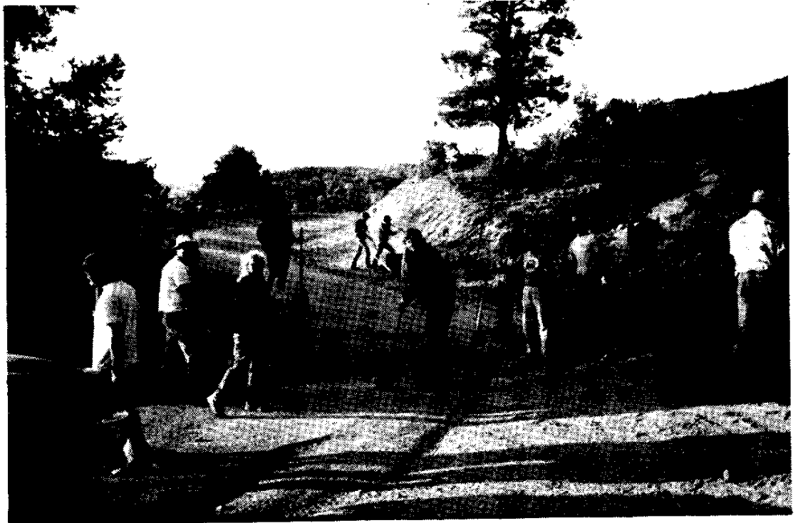
The hole in the Alamar Mtn. Road is almost filled in.
